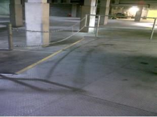
Chain edge protection is often not replaced and drops down at the centre point providing poor protection.
